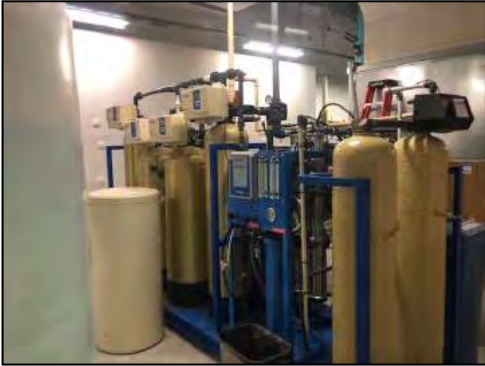
4 th Floor Mechanical Penthouse
