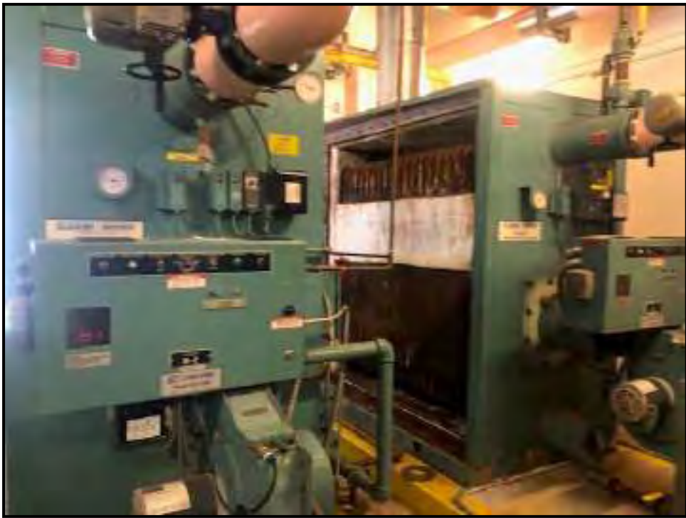
4 th Floor Mechanical Penthouse
